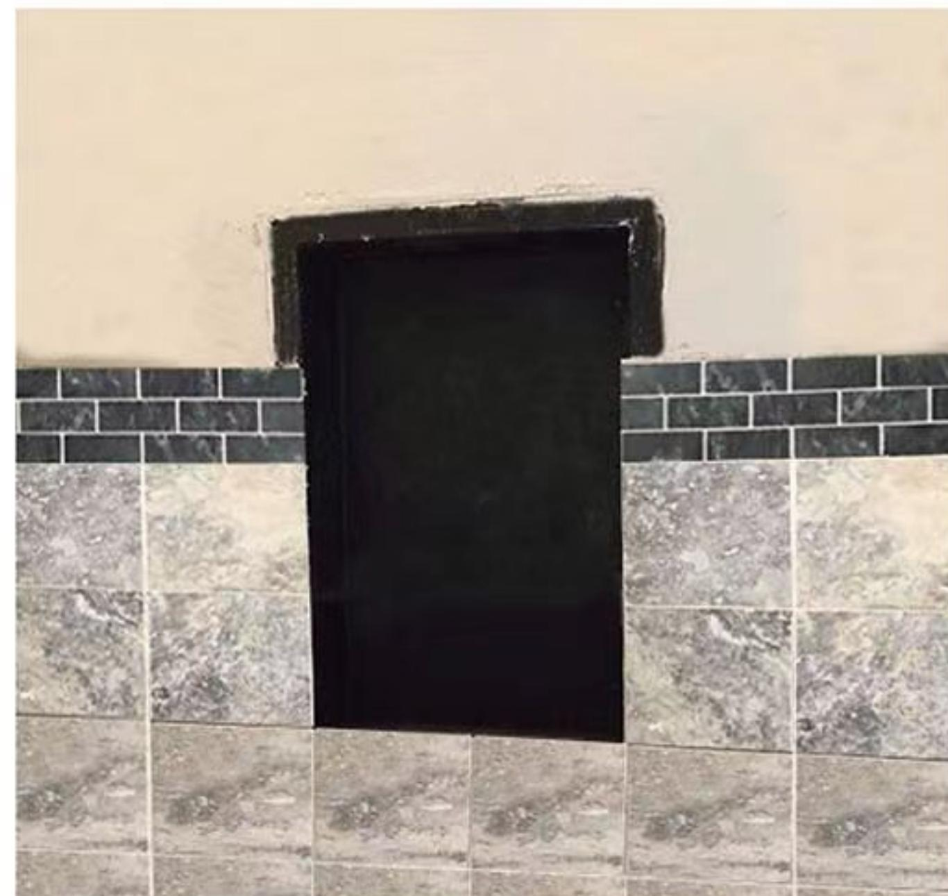
Step 3:Skim a coat of polymer modified thin-set mortar around the edge of the niche to feather out the flange to the substrate.
