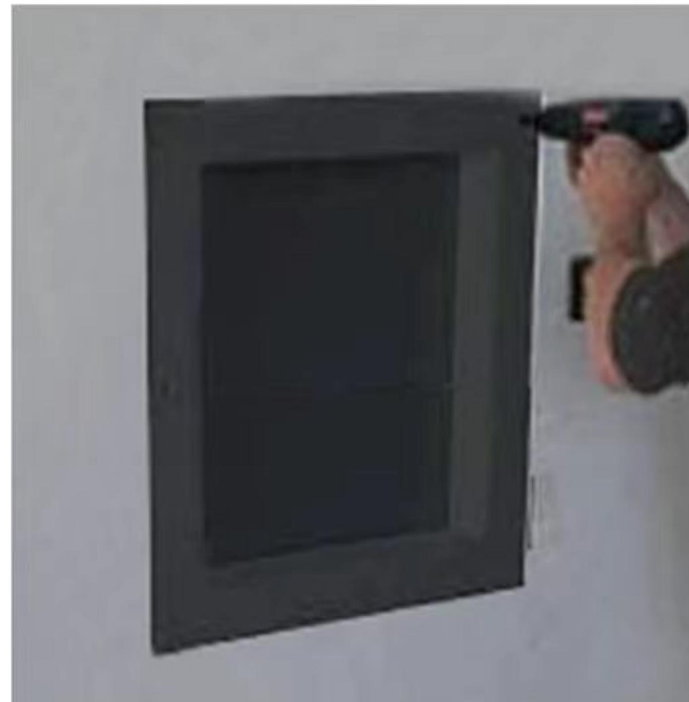
Step 2:Add a continuous bead of adhesive caulk on the back of mounting flange and secure it to the wall cavity with wall fasteners(fasteners not included, galvanized roofing nails may be substituted).A power screwdriver may be used if a low resistance setting is available ,otherwise,tighten all fasteners by hand and don't over tighten!
